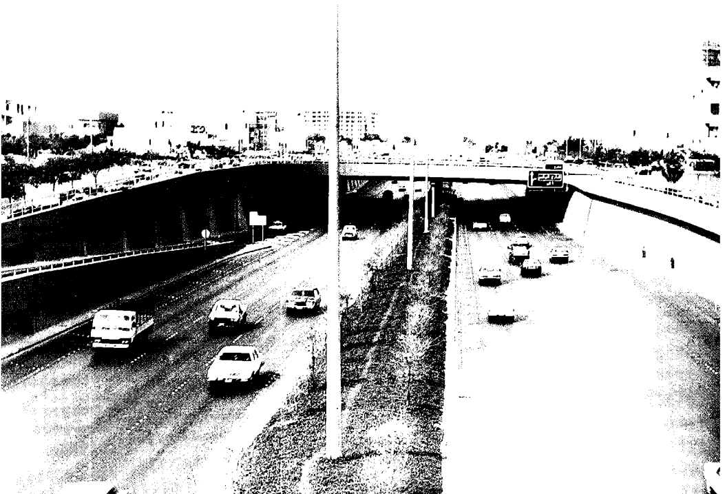
Tunnels and bridges.
