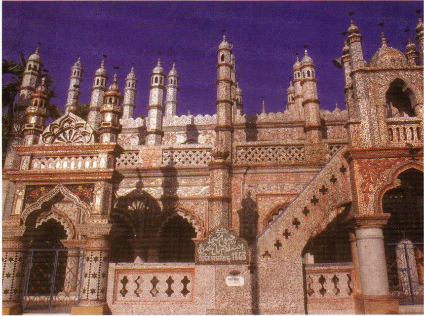
The historic Chini Mosque at the northern district of Nilphamari Constructed in 1863
