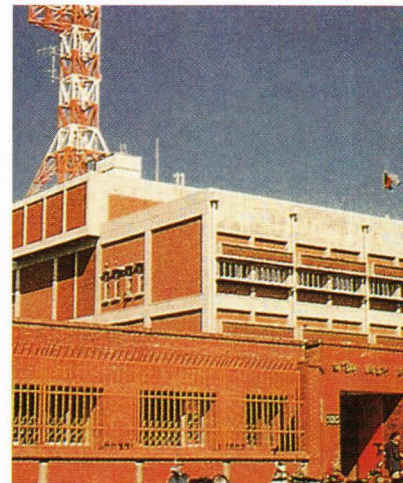
A view of Bangladesh Betar (Radio) building in Dhaka
